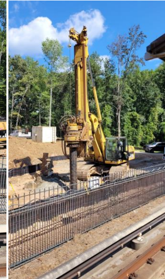
North/ South Property- Foundations for Bridge
